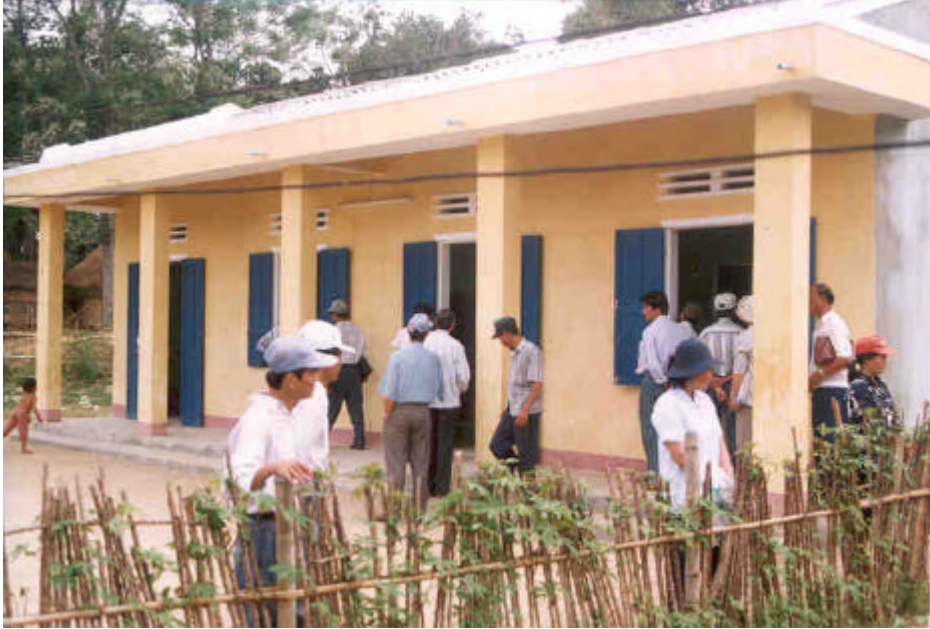
Figure 4. The new school of the Ten village in Quang Ngai after the three year project.
